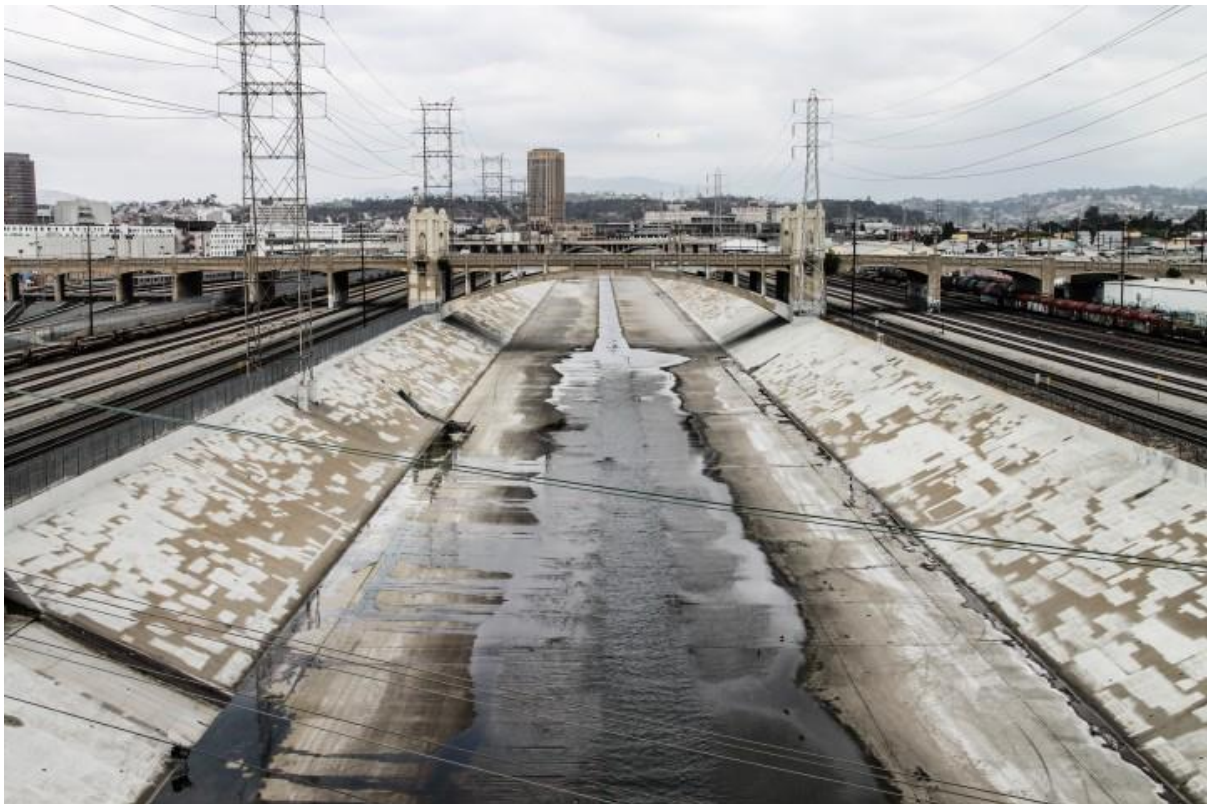
Figure 1: Extreme modification of catchments leads to complete loss of ecosystem services, reduction in habitat functionality, and may result in complete destruction of aquatic and other associated habitats.
