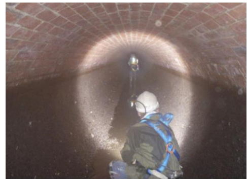
Fig. 2 Zebra mussels encrusting Yorkshire Water water pipes
