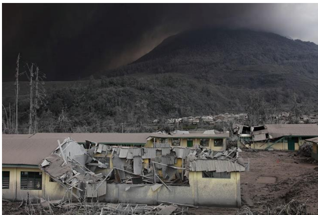
Figure 1. Partial roof collapse of a school in a village which has experienced heavy ash fall from Sinabung volcano, Indonesia, Jan 2014. Image taken by Dr Richard Roscoe and available on www.photovolcanica.com
